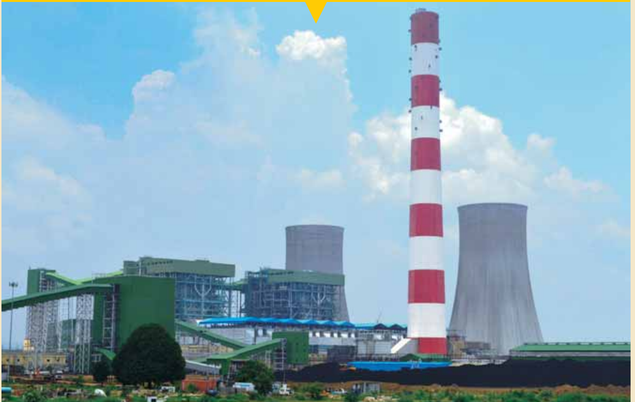
1320 MW Jaypee Nigrie Super Thermal Power Project, Nigrie, Madhya Pradesh
